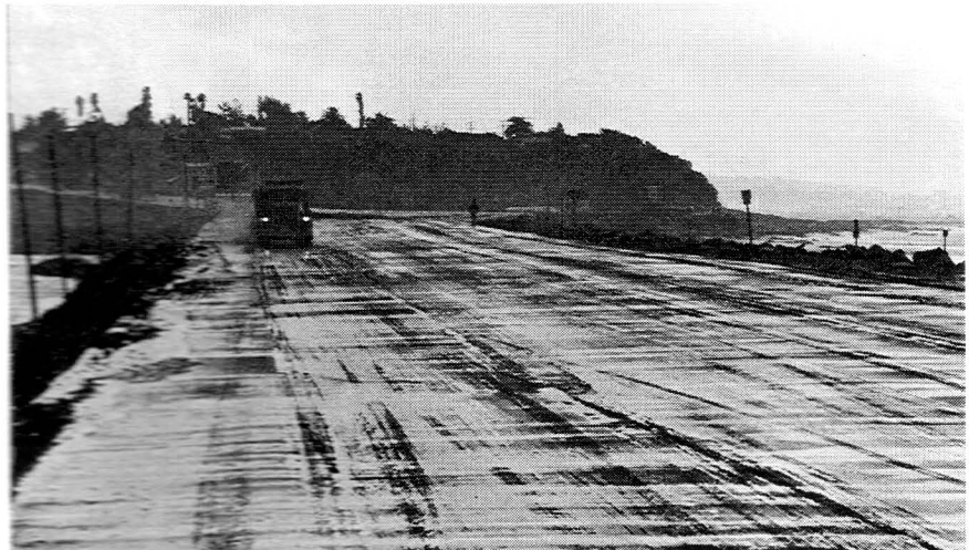
Aftermath of surf washing over Highway 101 in South Cardiff. Washouts along the highway are worsened by the loss of beach sand.
